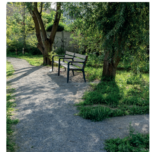
Parkpaden in halfverharding Park Oude God © Stramien cv
